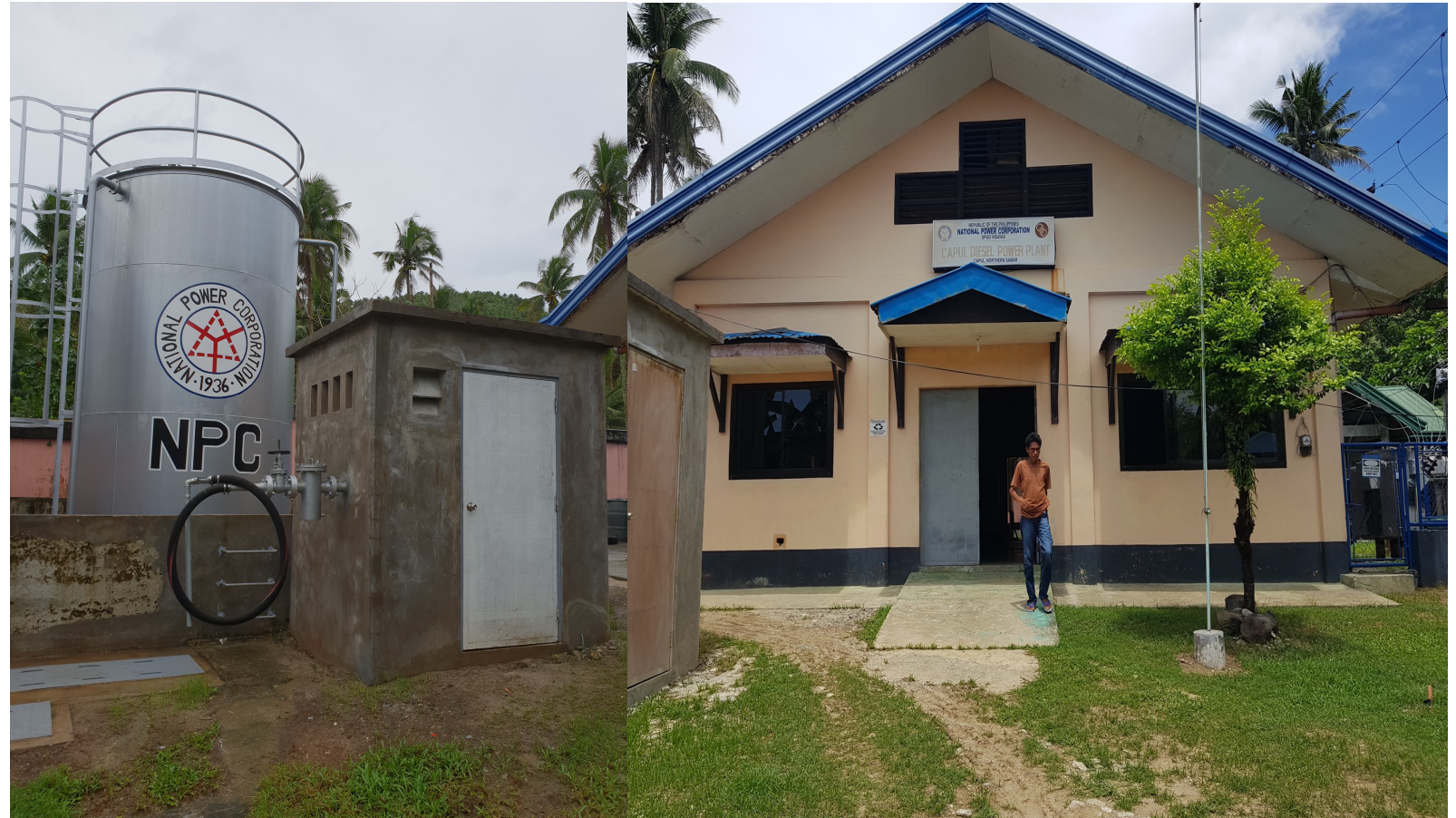
Capul Diesel Power Plant
