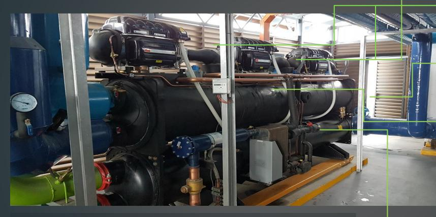
Danfoss Turbocor magnetic (maglev) intelligent compressors (3 units per chiller)
