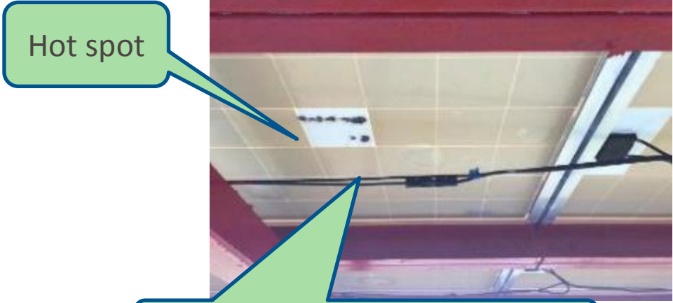
Cables not fixed nor supported
