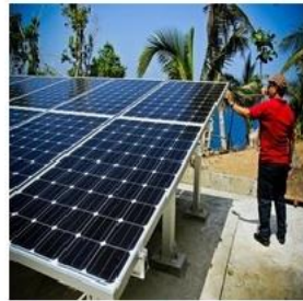
Cobrador Island Solar-Diesel Hybrid System
